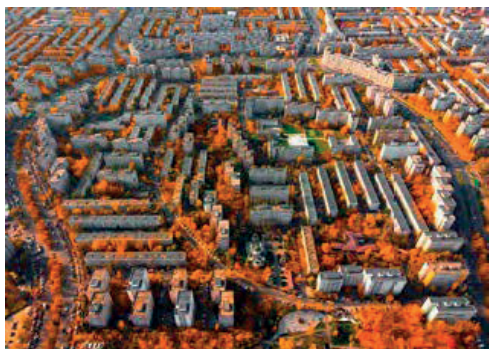
Figure 25. Drumul Taberei, 2022 (photo: Andrei Gherasim in INTI, 2024b)
