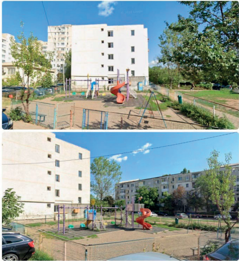
Figure 3. Assessment of the existing playground conditions
