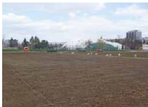
Figure 1. Collecting debris (stones, boulders, glass)
